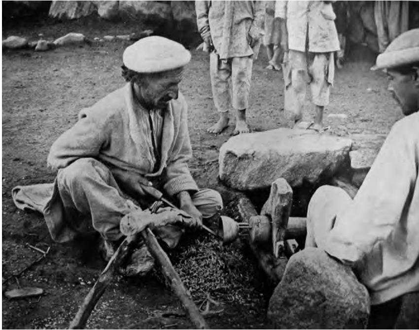
Figure 7: Traditional bowl turning in Hunza valley. After Lorimer 1938 Pl. IV.
