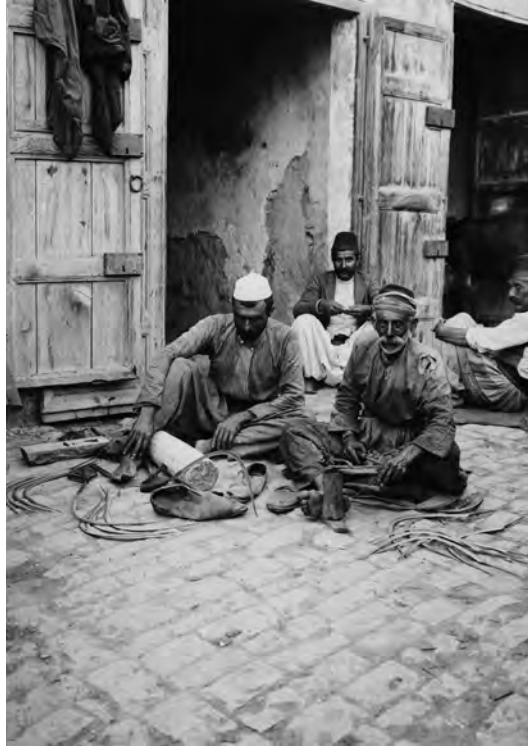
Figure 4: Blacksmiths in Nazareth serrating sickles (Matson collection).
